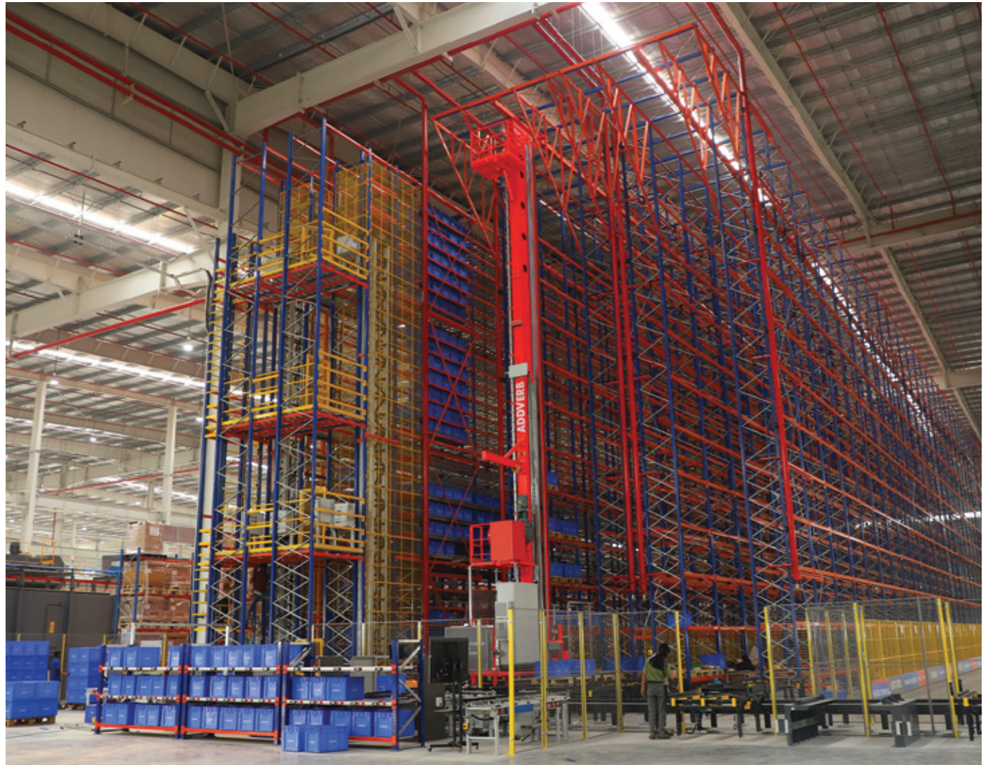
*Automated Storage and Retrieval System at Bot-Verse facility
